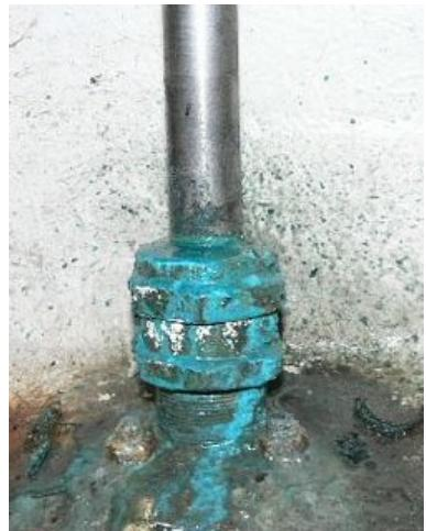
Then bring back the locking nut to the carrier and lock both carrier and lock nut together don't over tighten the joint as it will eventually need to be re-packed again at a later date. There is very little room under the
